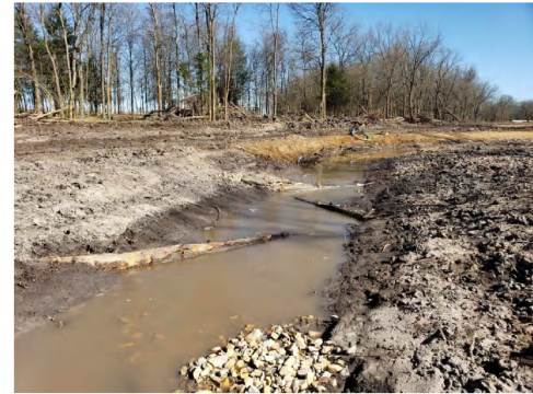
CONSTRUCTED LOG RIFFLE CONSTRUCTED FEBRUARY 2019
